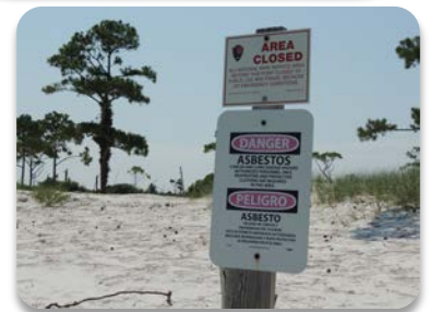
Due to years of weather and beach erosion, asbestos-containing building materials had scattered across the beach, resulting in asbestos fibers impacting beach sand.
