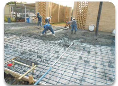
Our design/build team engineered and constructed onsite pollution control facilities.
