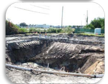
Primary remedy included dewatering and excavating over 30 feet below land surface.
