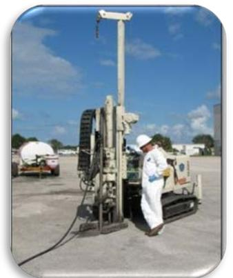
*EVO delivery completed at specific subsurface intervals using direct push technology.*
