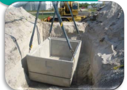
The project team self-performed all system component installations.
