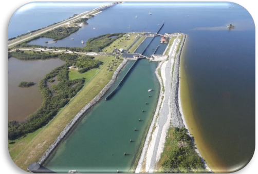
Aerial view of Canaveral Lock, January 2, 2020
